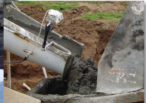
This camera mounted on the chute allows Vulcan's drivers to stay clear of concrete pumps.
